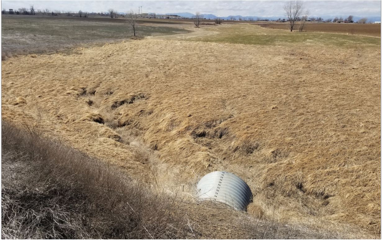
Photo 7 - Overview of DP3 and Drainage 2 upstream of culvert in the southeastern portion of the project area. View is to the southwest.
